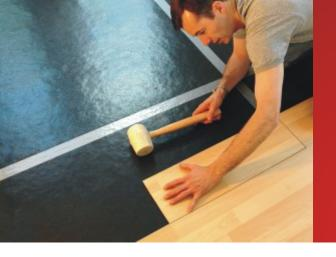
QuietDown is a multi-purpose, highperformance acoustic underlay engineered from recycled rubber to reduce sound transmission through subfloors.
